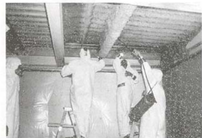
Typical high risk abatement project
